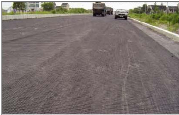
Figure 6. Reinforcing retaining walls and embankments Figure 7. Reinforcement in repair of deteriorated asphalt surfaces
