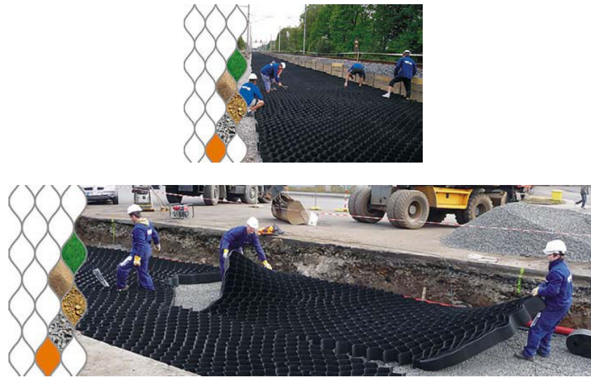
Figure 5. Installation Sacco structure
