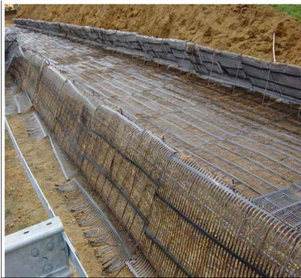
Figure 6. Reinforcing retaining walls and embankments Figure 7. Reinforcement in repair of deteriorated asphalt surfaces
